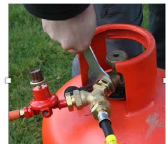
9. Use the spanner to tighten the fixings on both cylinders. Make sure they are firm. Do not over tighten.
